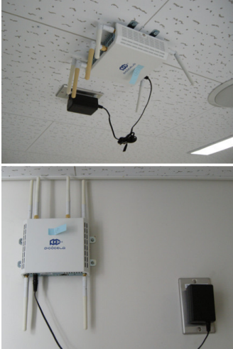
Fig. 6. PCWLs installed on the ceiling and wall
